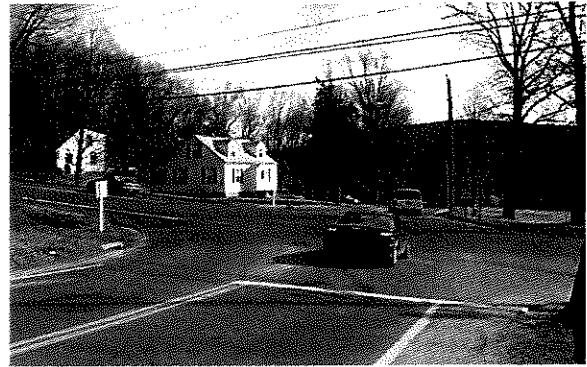
Poor Sight Distance at Route 190, Gulf, and Turnpike
