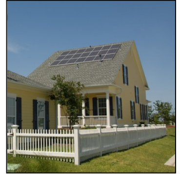
Residential solar panels
