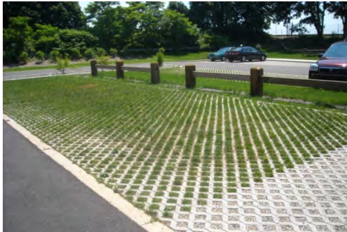
Example porous pavement treatment. Source: CTDEEP
