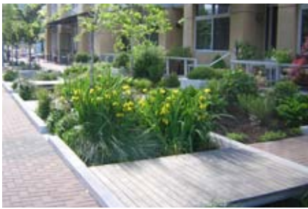
Permeable pavement and swales are part of the stormwater management plan for Portland's South Waterfront. Lush plantings are possible without watering maintenance. photo: Nevue Ngan Associates
