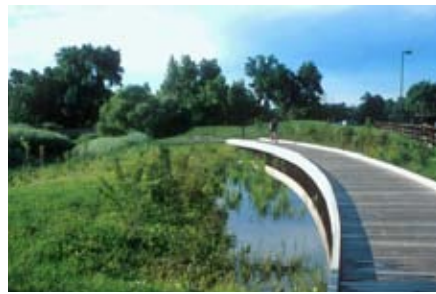
This constructed wetland near Denver, CO manages all of the surface runoff from an adjacent parking lot. photo: www.werf.org/livablecommunities
