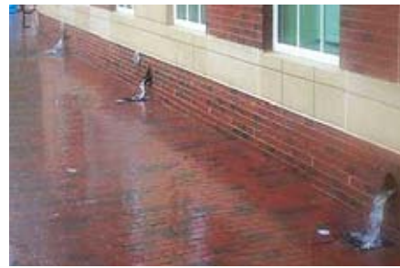
Rams Head Plaza at UNC Chapel Hill features an underground cistern. Above, downspouts convey roof runoff into the plaza inlets. The water is stored and later used to irrigate plaza plants. photo: http://sustainability.unc.edu
