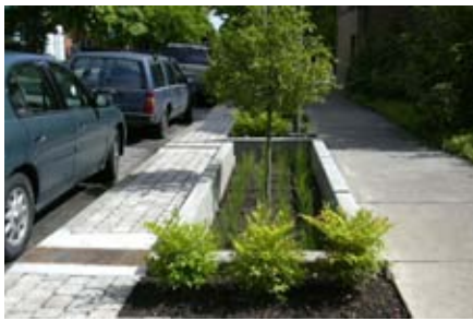
Stormwater infiltration planters in use in Portland, Oregon at Southwest 12th Avenue Green Street. The above image shows a newly installed planter in dry conditions. photo: Kevin Robert Perry
