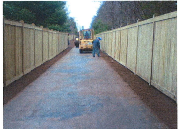
Rail-trail under construction in Simsbury
