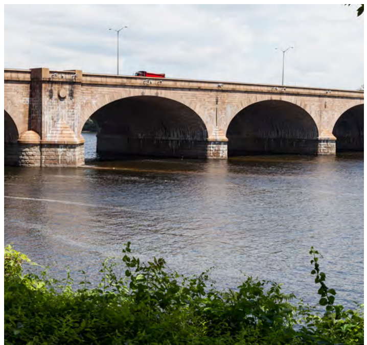
Figure 03.10 – The Bulkley Bridge between Hartford and East Hartford
