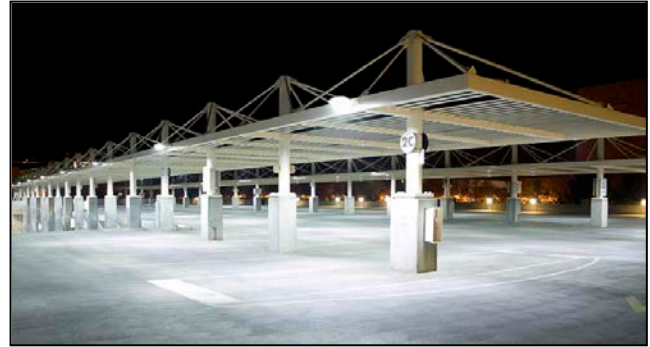
Parking lot lighting
