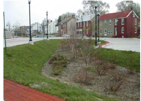
Example bioretention area 12 .
