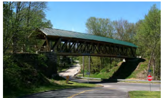
Hop River Trail bridge over Route 316, Andover
