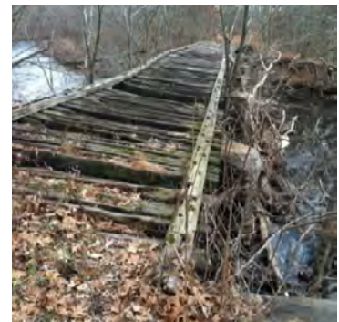
Existing Bridge over Hop River near Kings Road.
