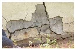
This is a reimbursement program for visual inspection and core testing for failing concrete foundations due to pyrrhotite.
