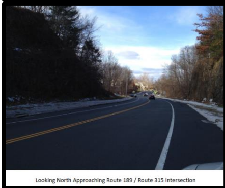
Looking North Approaching Route 189 / Route 315 Intersection
