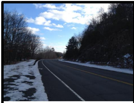
Looking South on Route 189 Near the Bloomfield / Simsbury Town Line
