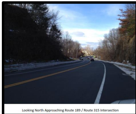
Looking North Approaching Route 189 / Route 315 Intersection
