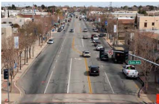
Lancaster Boulevard before Complete Streets redesign
