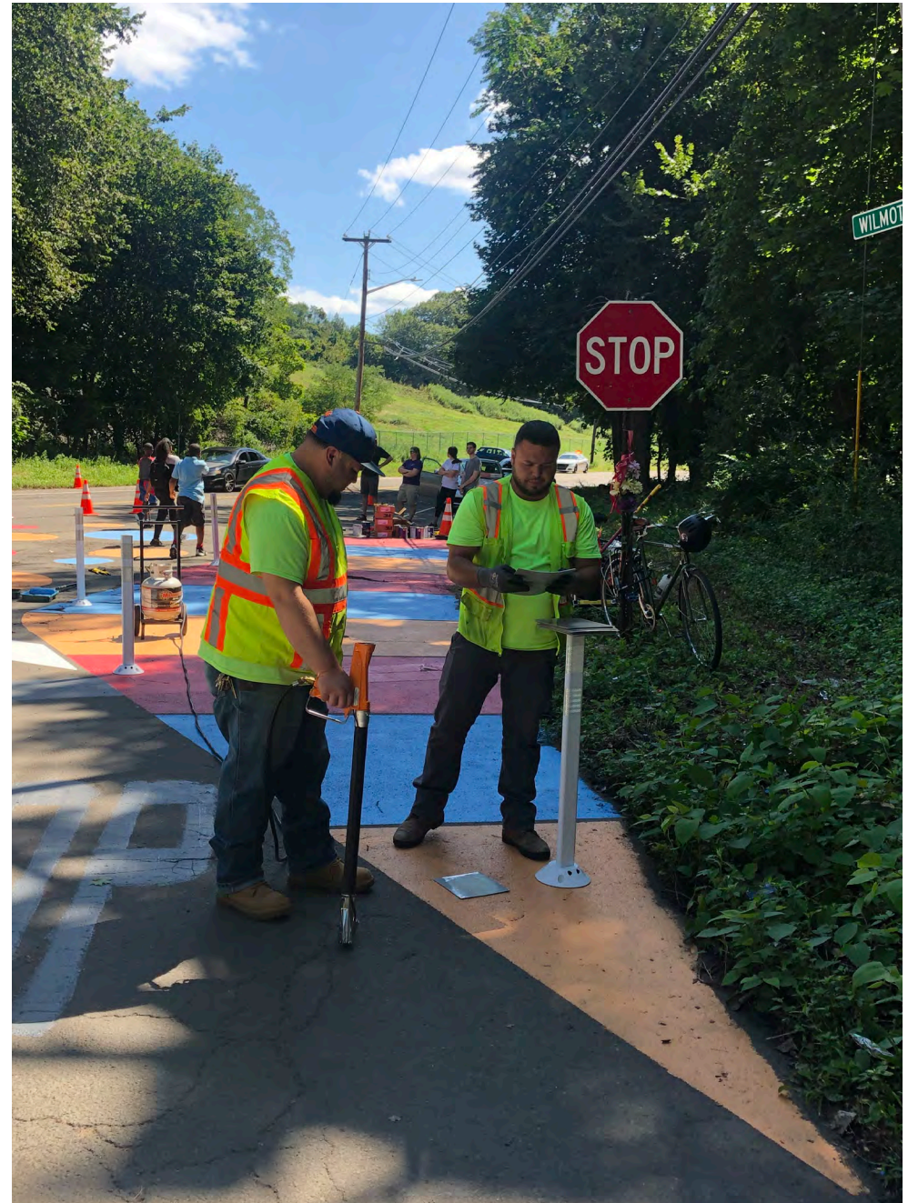
Advanced coordination with New Haven's Department of Transportation ensured trained professionals could properly install vertical delineators while volunteers painted curb extensions and crosswalks. Photo: Street Plans
