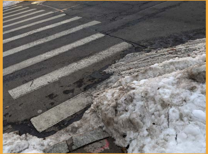
Lack of snow removal has rendered this curb ramp inaccessible to wheelchair users.
