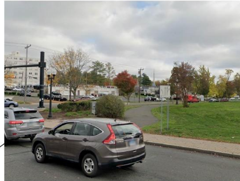
The intersection with Trout Brook Dr includes a connection to the Trout Brook multi-use path
