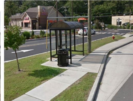
Walnut Street bus stop location has a sign, shelter with bench, and a trash can
