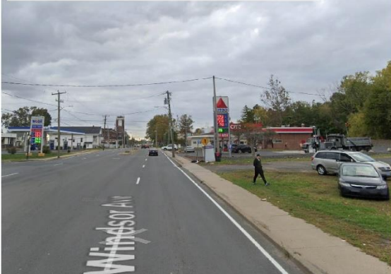
The sidewalks along Windsor Ave at the northern end of the corridor do not have a buffer between the sidewalk and the road
