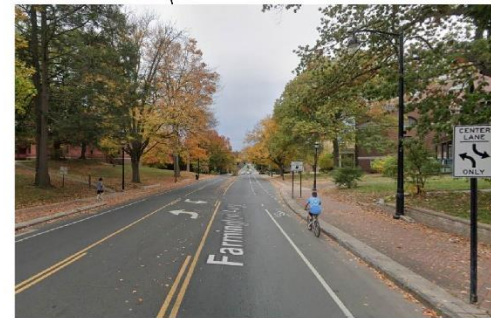
In the center portion of the corridor, the four-lane roadway transitions to a two-lane road with a two-way left turn lane and bike lanes in each direction
