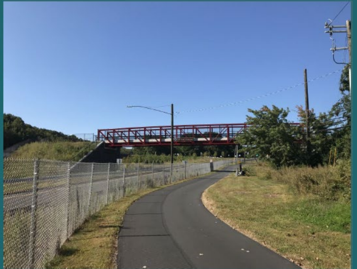
I-384 Exit Overpass in Bolton, CT
