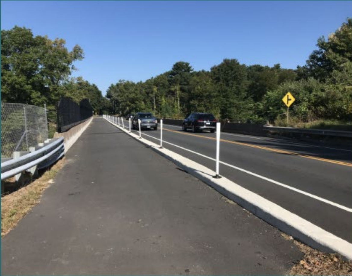
Roadway-level 2-way Cycletrack in Bolton, CT
