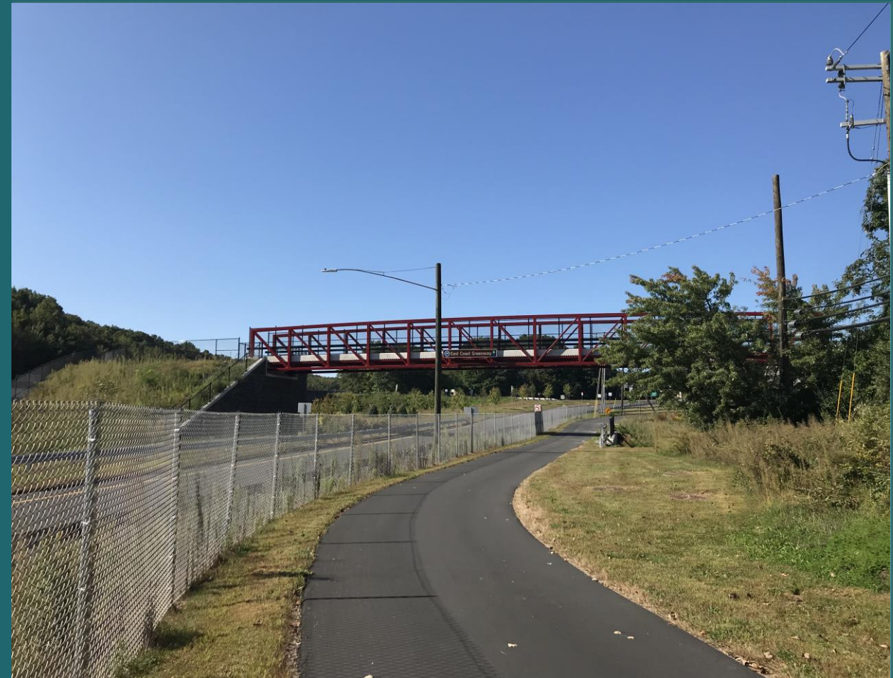
I-384 Exit Overpass, Bolton, CT
