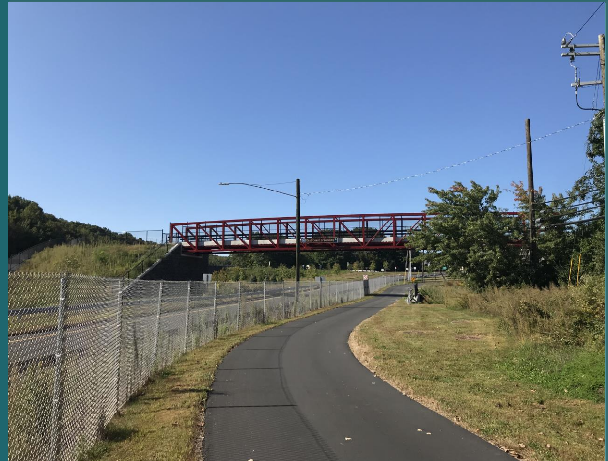
I-384 Exit Overpass, Bolton, CT
