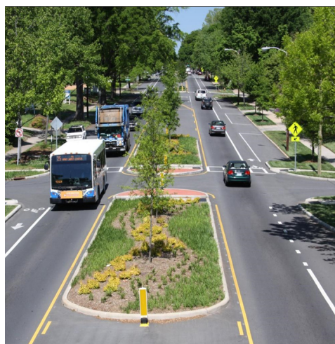
Example of a road with a median and pedestrian refuge islands. Source: City of Charlotte, NC
