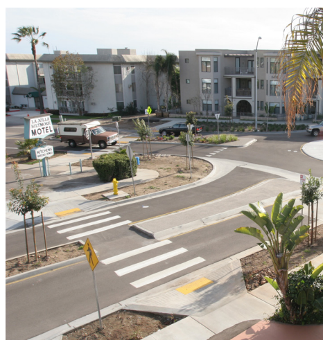
Median and pedestrian refuge island near a roundabout. Source: www.pedbikeimages.org / Dan Burden
