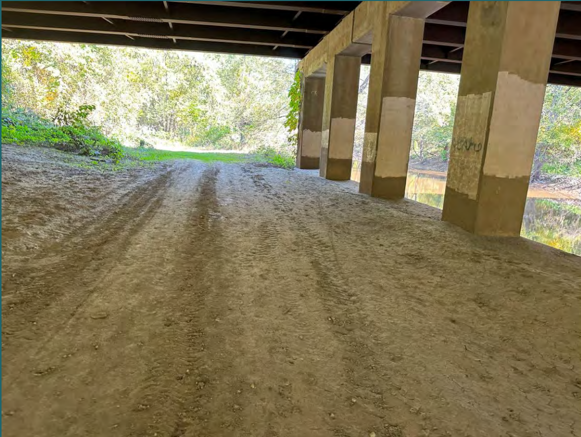
Hockanum River Trail under Rte 2 overpass. View looking east.
