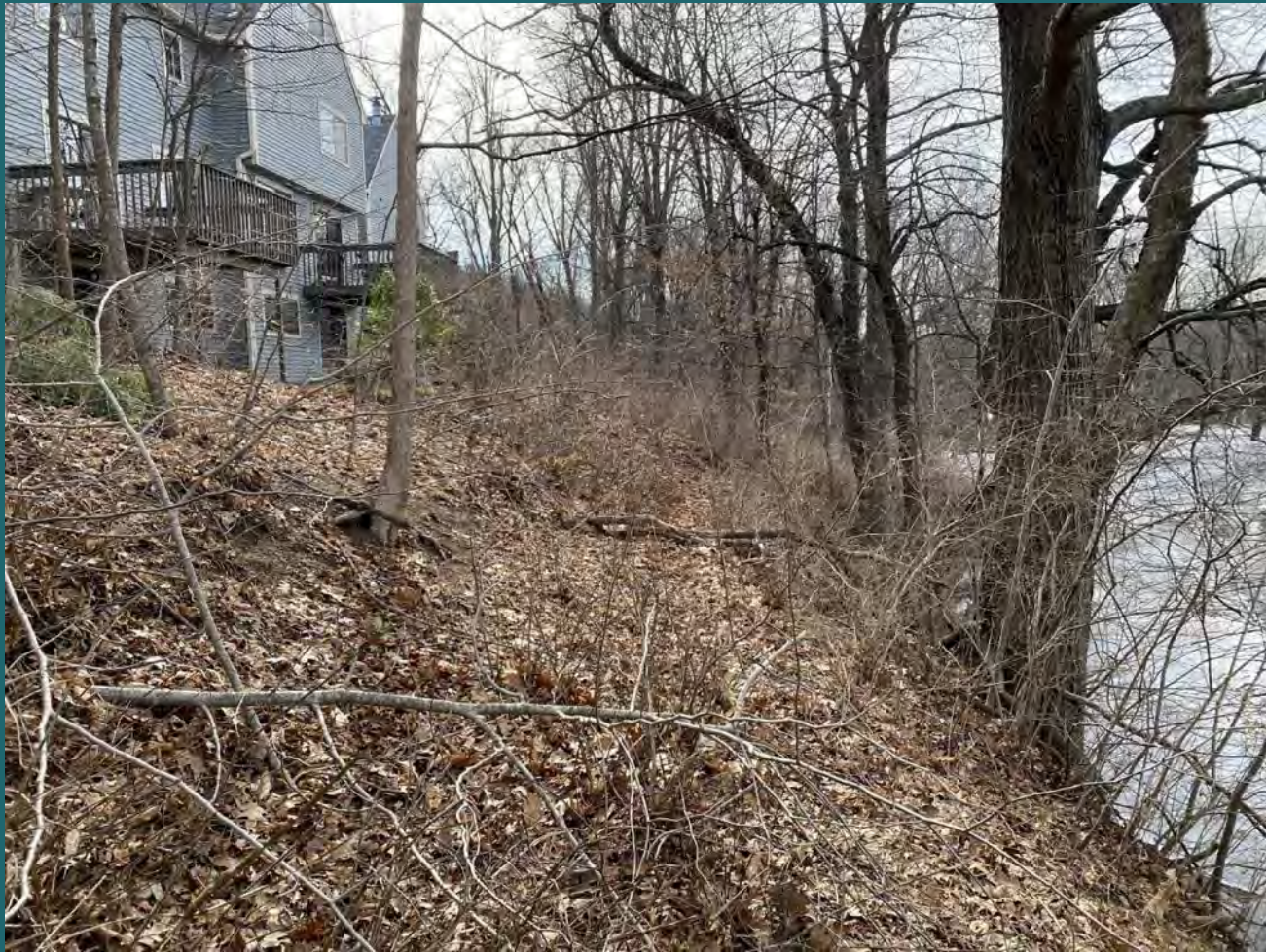
Farmington Riverbank Current Conditions
