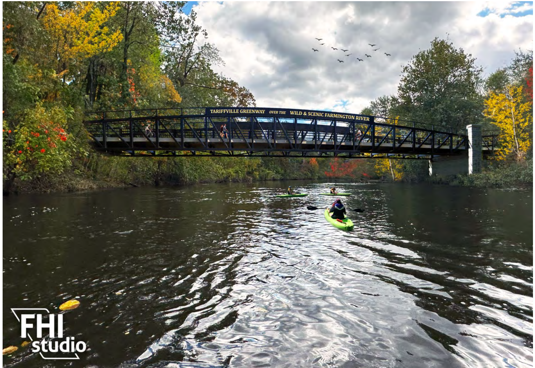
Exhibit 1-6: The future trail crossing of the Farmington River offers the opportunity to create a memorable landmark for the ECG in Simsbury
