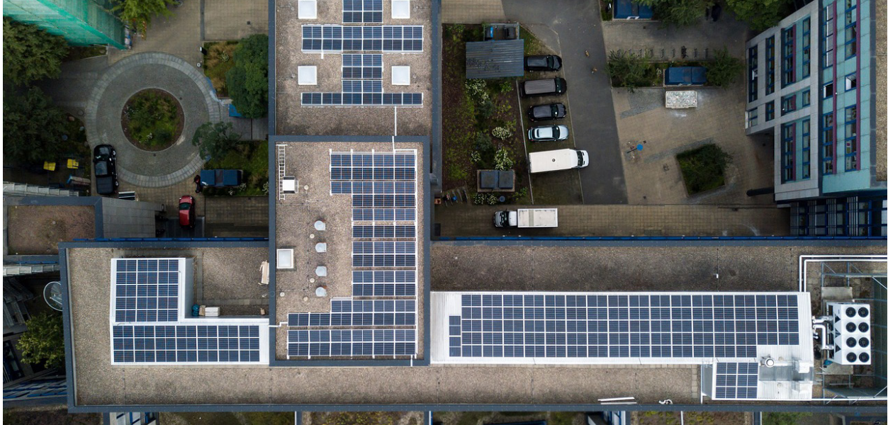
Figure 34: Aerial view of rooftop solar panels on a building.
