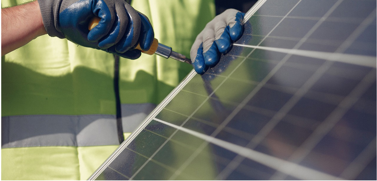
Figure 32: Worker installing a solar panel.
