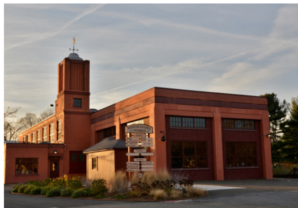
Figure 12: The historic Witch Hazel Plant in Essex, CT.
