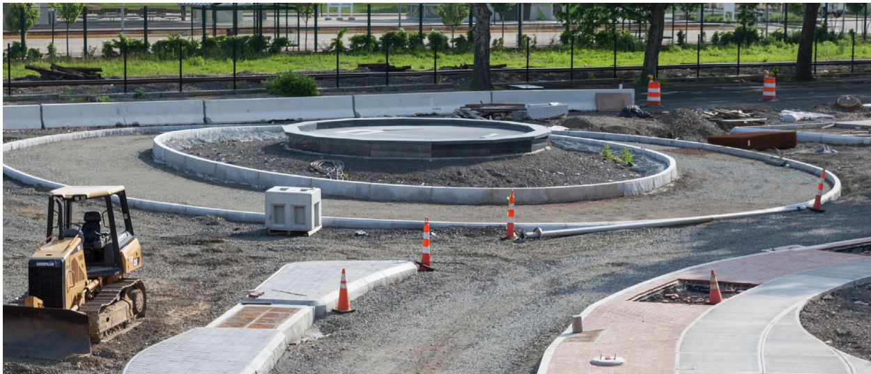
Figure 39: Construction of a roundabout in New Britain, CT.
