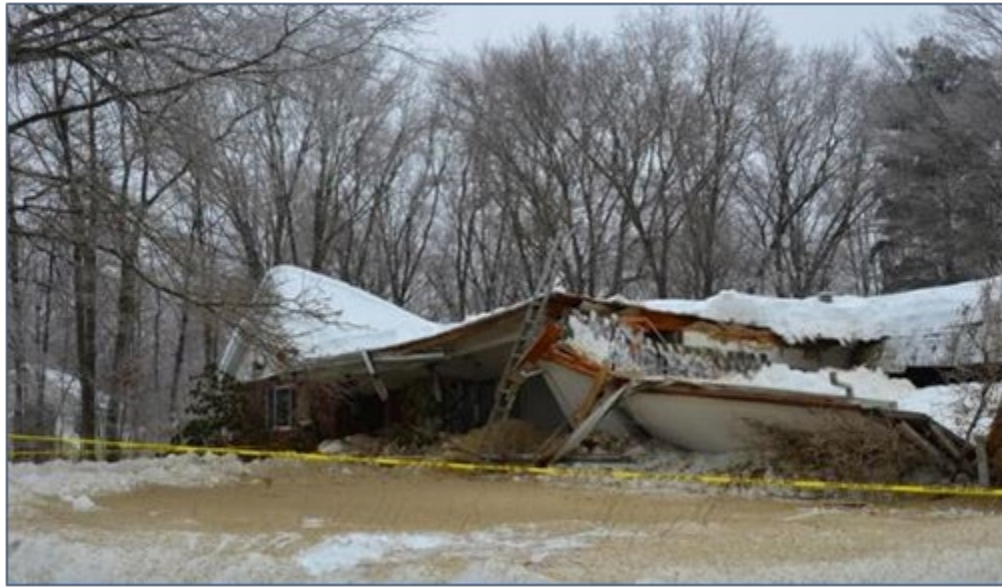
Hebron Building Collapse due to Heavy Snow Loads, February 2, 2011 Credit: John Sholtis, WTNH.com
