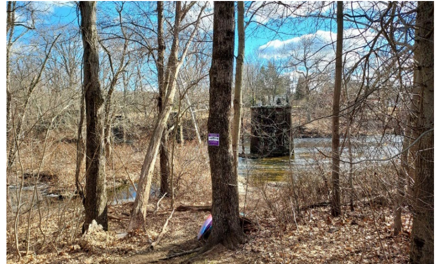
Exhibit 3-1: Abandoned rail abutment north of Tariffville Park crossing north towards Route 189 (Exhibit 3-3, Location B)
