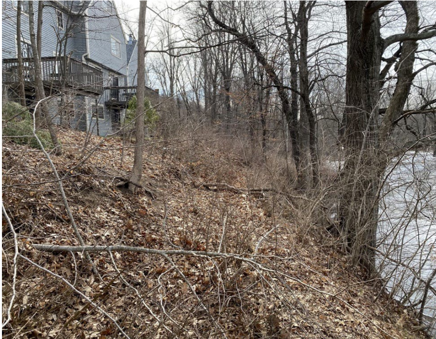
Exhibit 4-8: Farmington Riverbank Existing Conditions, photo view facing southwest/upriver
