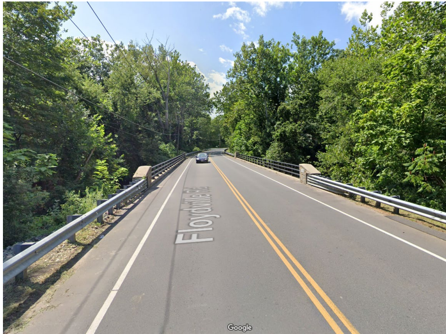
Exhibit 4-12: Existing Floydville Road bridge across the Salmon Brook (Source: Google Maps Streetview)
