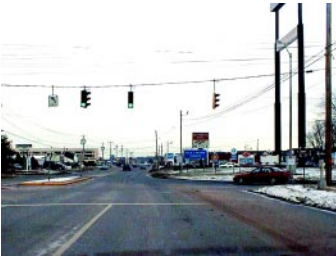
Route 75 at Route 20 Westbound
