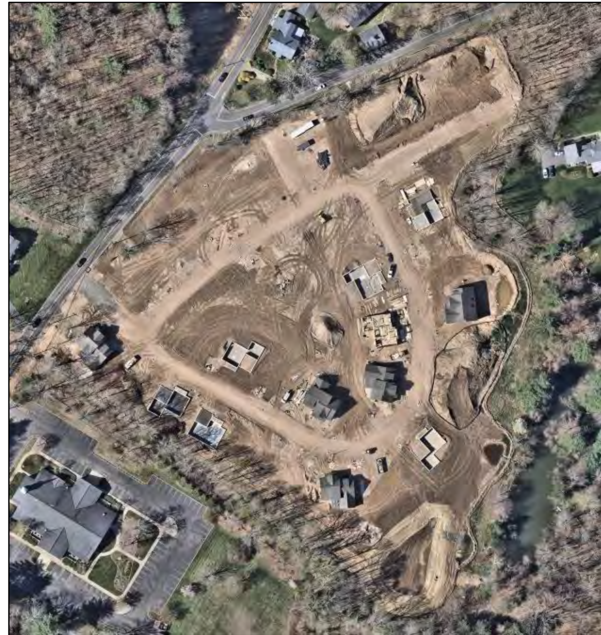
Applegate Village under development. Source: NearMap imagery from April 2024
