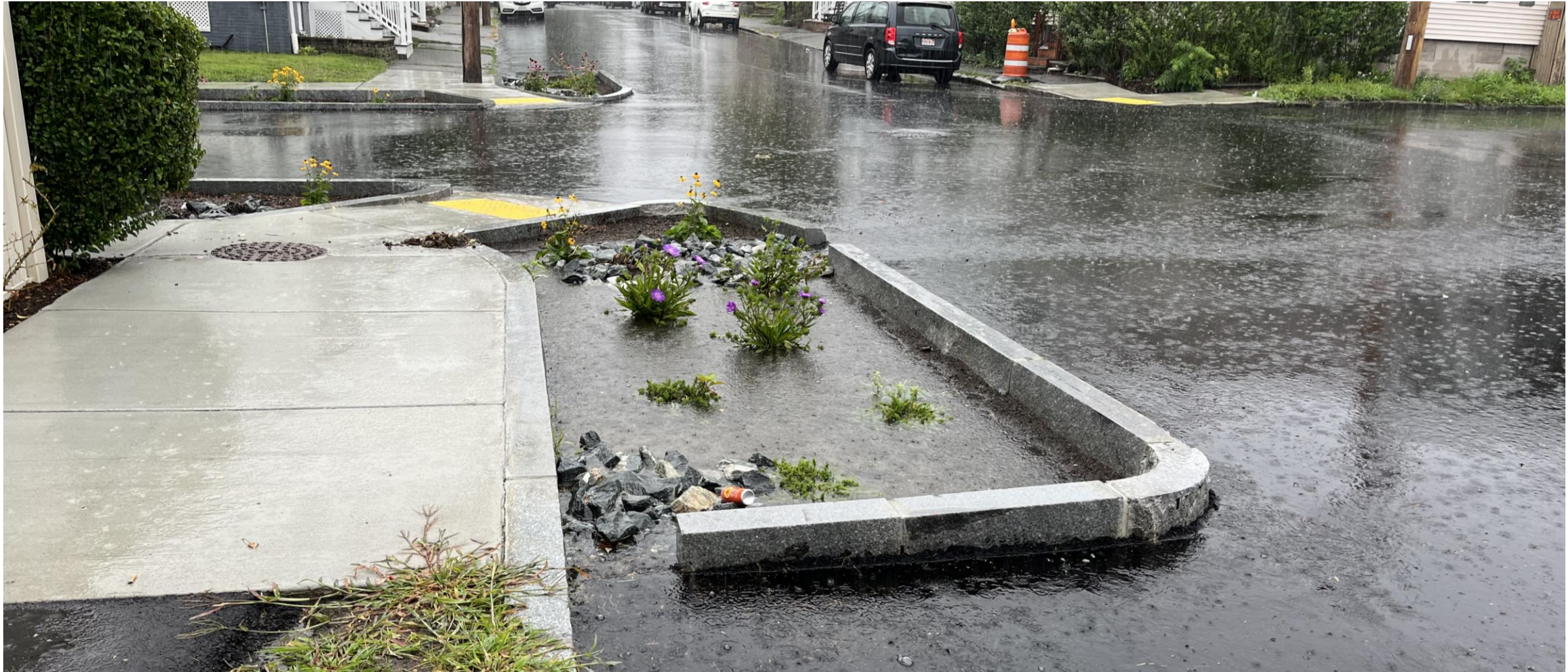
Photos: Barry Park Project in Lynn, Massachusetts, Weston & Sampson
