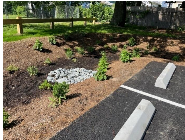
A bioretention basin in Lynn, MA designed by Weston & Sampson
