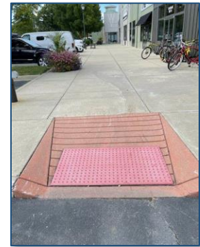
Figure 4: An example of an ADA-Compliant curb ramp at a crossing point.
