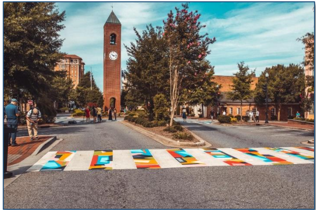
Figure 6: a crosswalk in Spartanburg, SC made highly visible through implementation of a crosswalk mural.
