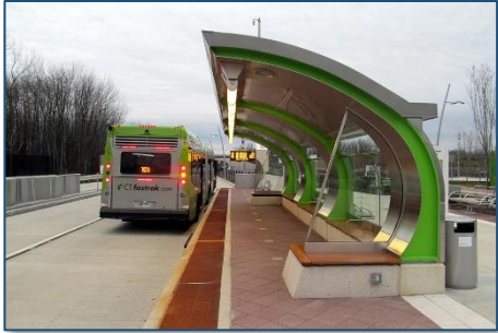
Figure 5:CT Fastrak station with curbside tactile warning strips.
