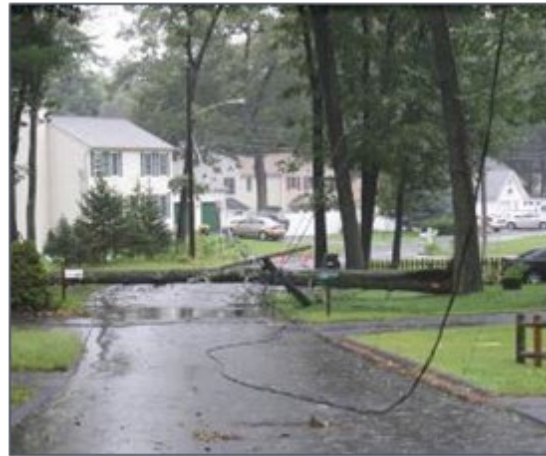
Downed Wires in Enfield after Hurricane Irene
