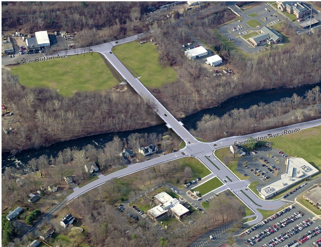
Source: Preliminary Design Phase Design Report Extension of Monteith Drive over Farmington River, AECOM, April 6, 2018
